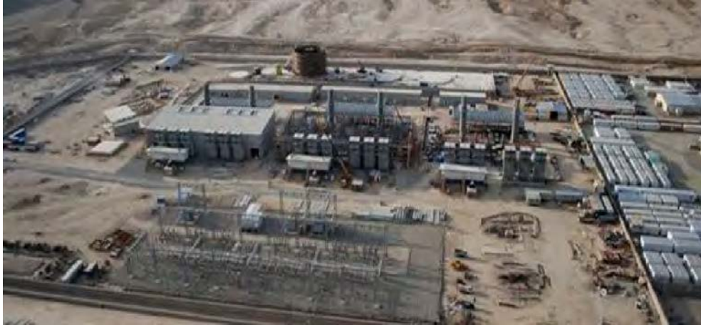
Photo of Tarakhil Power Plant, from SIGAR report, August 7, 2015
